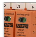
green protector status indicator light – insert in working order red – to be replaced
